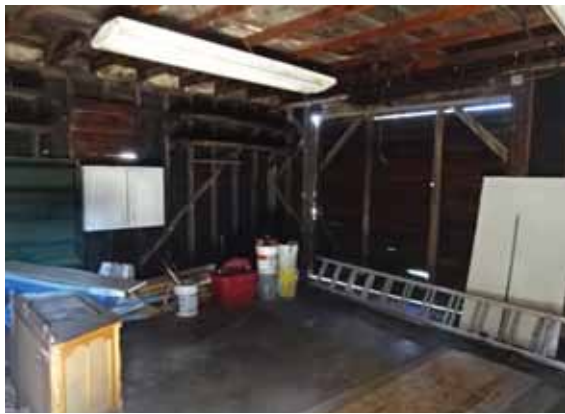
Interior view of the storage building.
