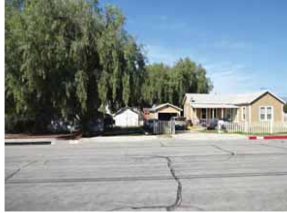
Eastern elevation of the central parcel viewed from North Cataract Avenue (Residential dwellings at 911 & 917 N. Cataract Ave. shown).
