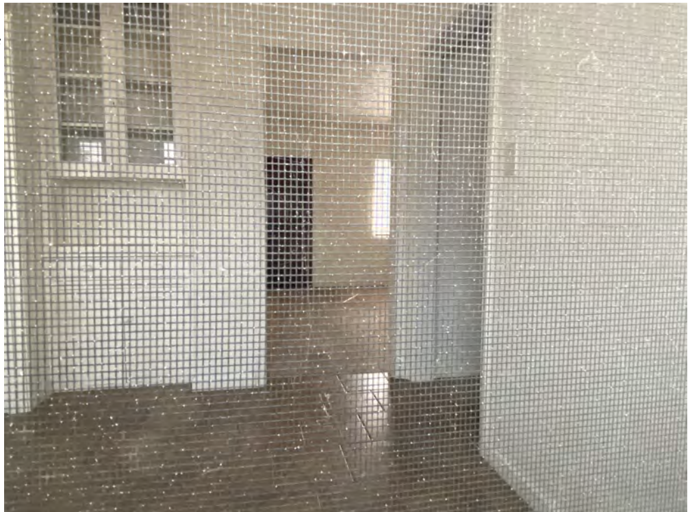
Photo 18: View looking through the window of 929 Cataract Avenue.
