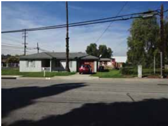
Eastern elevation of the southernmost parcel viewed from North Cataract Avenue (Residential dwelling at 907 N. Cataract Ave. shown).
