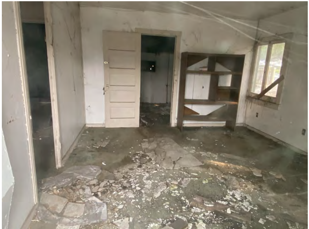
Photo 14: View through the window 911 Cataract Avenue.
